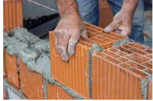
Figure 2 Hollow Clay Block
